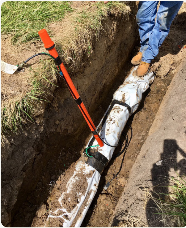
Properly installed V-Bio® with test probes.
